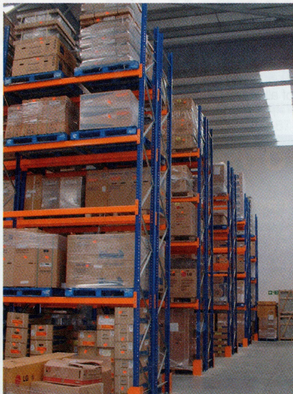
Wave Air Conditioning's new warehouse at Basingstoke
